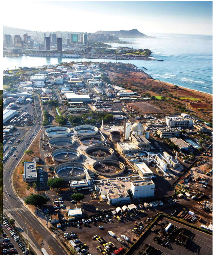
Sand Island 100 mgd WWTP, Hawaii
